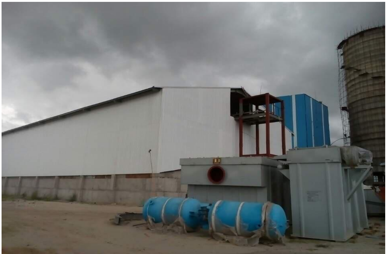
Bengal Cement Factory-Material Shed, Barodi, Narayangong.
