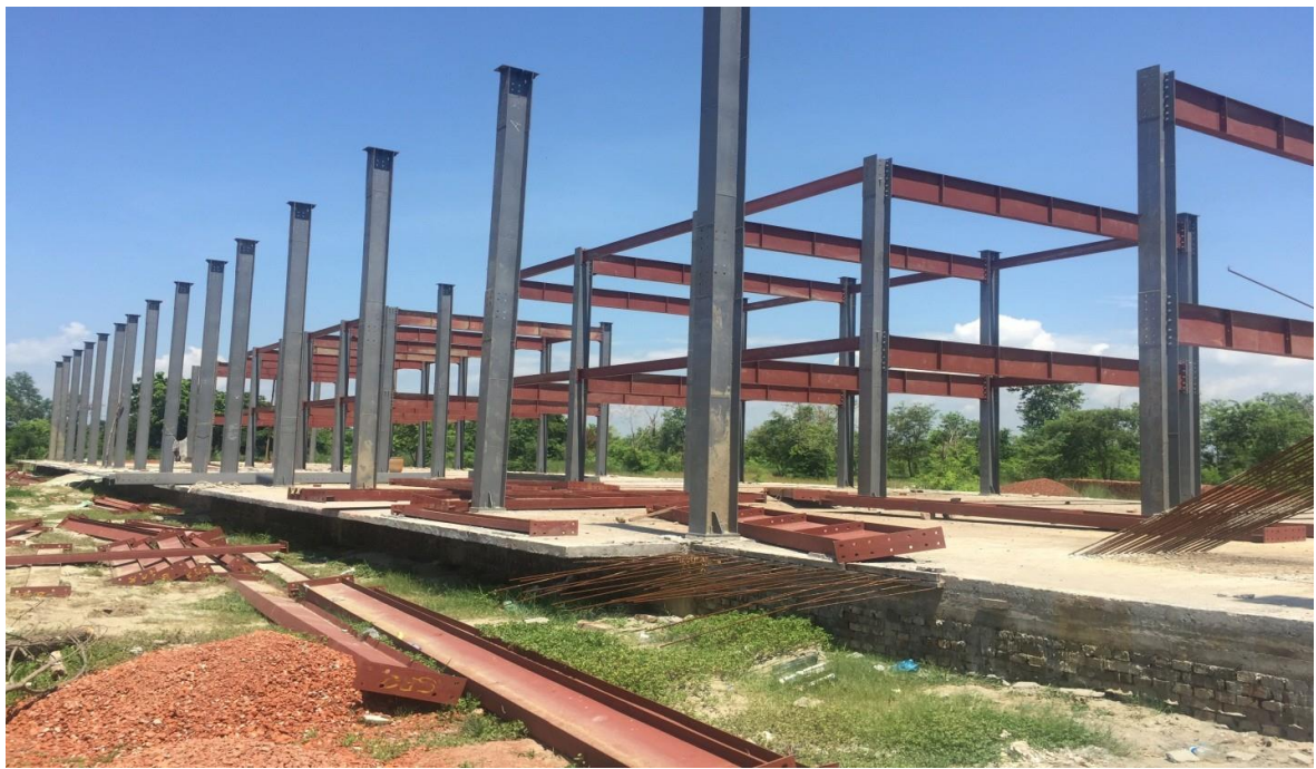
Hamdard University Hostel Building (MeghnaGhat, Munshigonj) Area= 65,000 Sft(Three Storied) (Complete)
