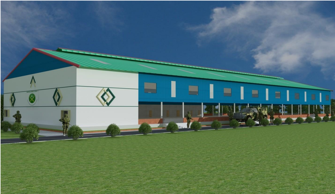
Multi-Purpose Shed (Chittagong Cantonment) Area= 44,500 Sft(Complete)
