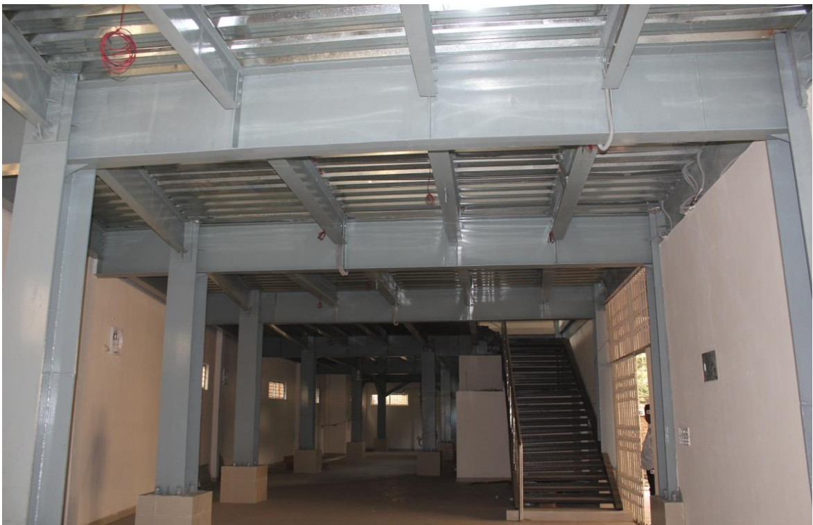
Hamdard Warehouse Building, Tejkunipara.(Complete)
