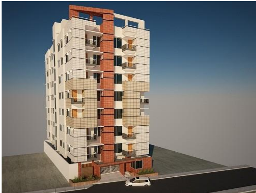
Abiding Noor Castle- 267/1, East Rampura, Dhaka =22,350 Sft (7th Storied) - (Complete)
