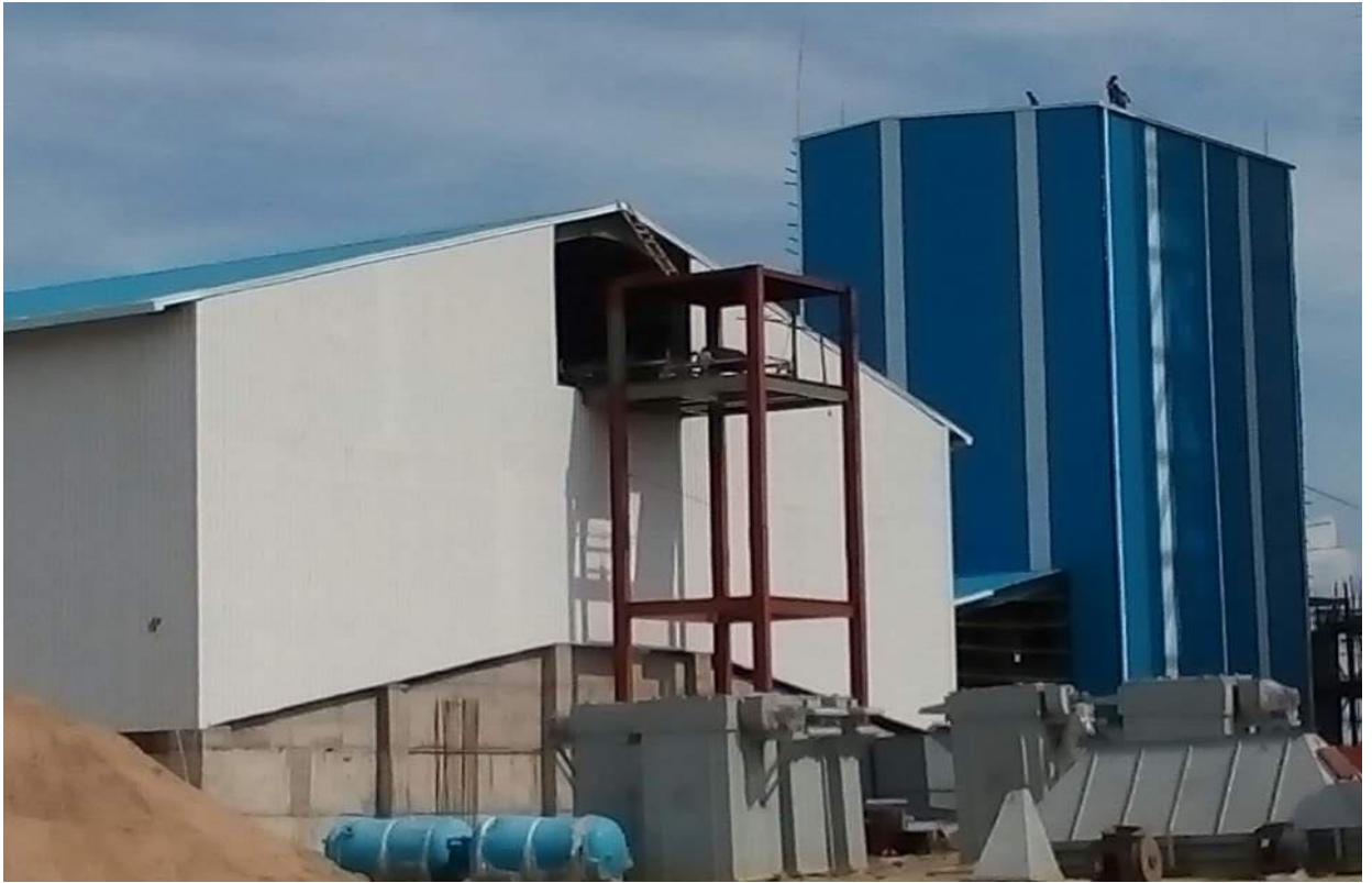
Bengal Cement Factory, Barodi, Narayangong.
